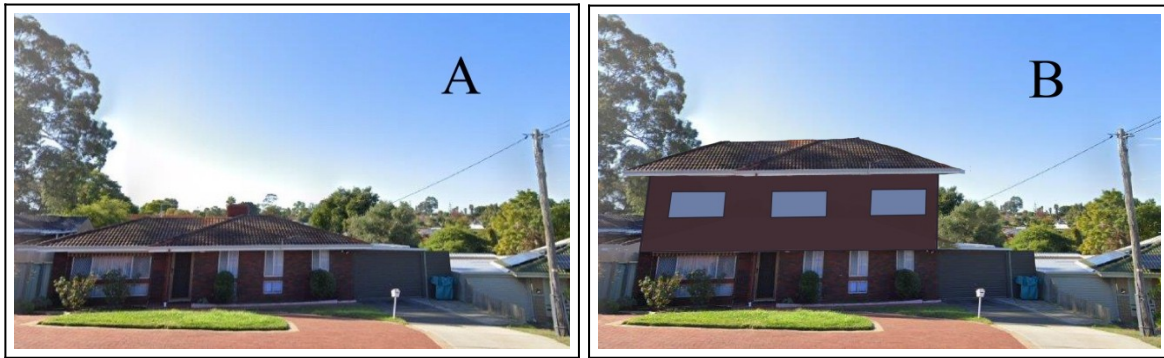
Figure 5: A common suburban 1 storey house (A), and with drop-on 2 nd storey added (B).
