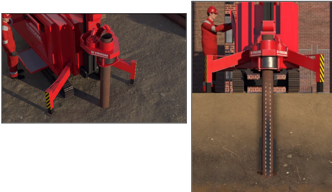
Figure 9. A couple of images of machine that can be used for the ‘steel pipe screw pile’ (Vroom, 2023)
